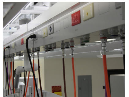
Overhead service carriers pre-plumbed and pre-wired supporting power, plumbing and lighting
