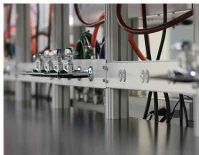
Manifolds to accommodate plumbed services, power and data
